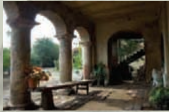
Interior del pasillo principal
